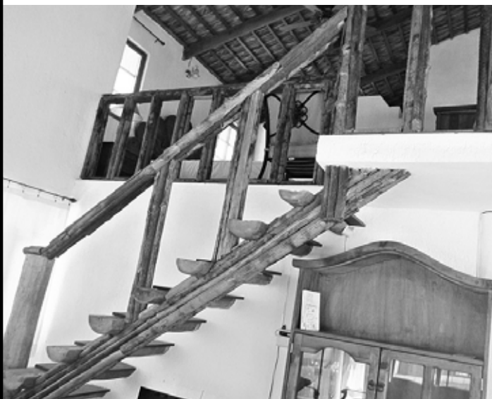
Casa 7 Living Room and Bedroom in Loft
